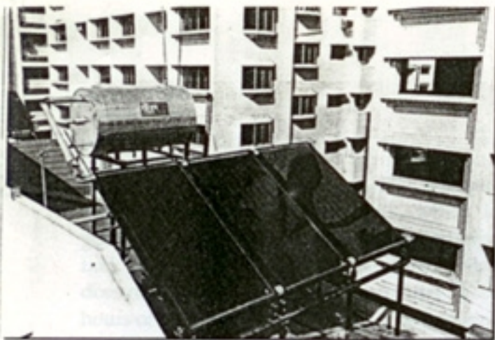
Pressurized solar heating system installed in a company in Pune.
